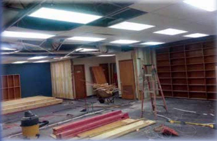
Remodeling of new building in Bryan, Texas
