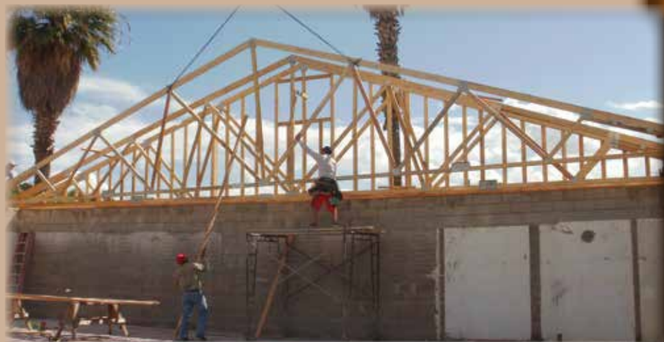
After workers gutted the old building, roof trusses go up in Nogales
