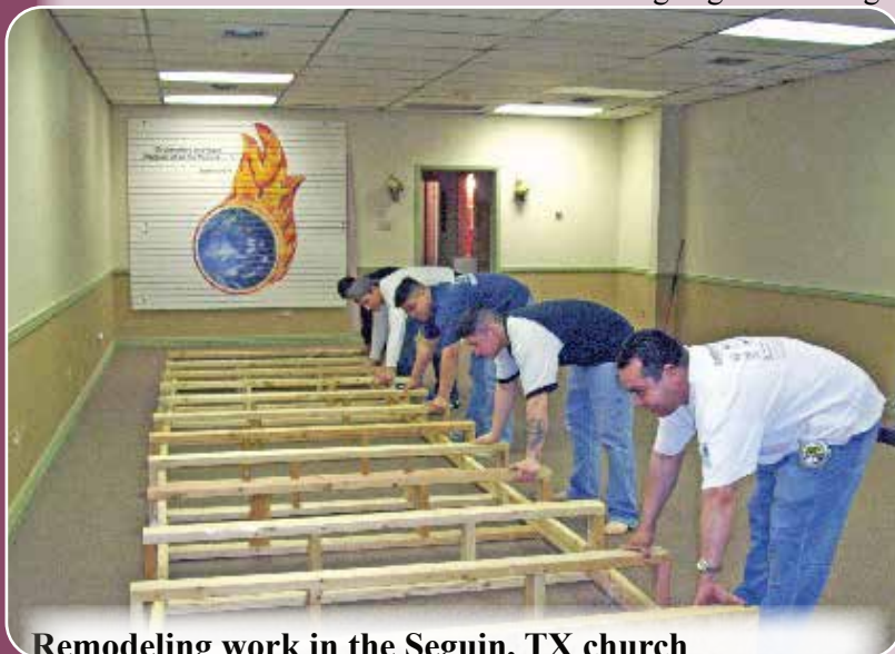
Remodeling work in the Seguin, TX church
